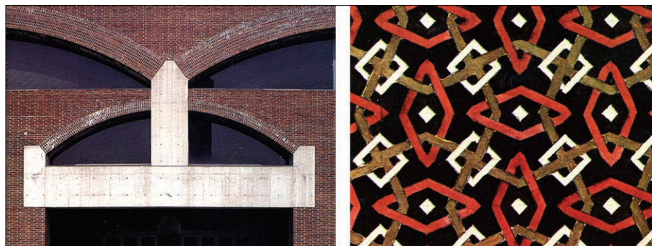
Figure 5 Defining structure and detail with colour contrast
